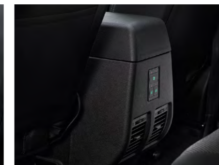
Control panel for air conditioning and heating
