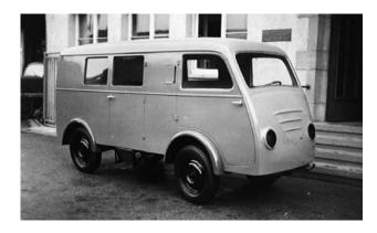
instead of a separate box body. As a result, BINZ created the first prototypes of a functional, plain and simple small box-body truck in 1949. The outer features of the prototypes differed from the Vischer cars by their one-piece windscreen and the three cross beads on the front of the vehicle.
